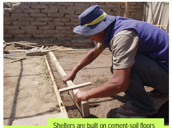
Shelters are built on cement-soil floors for better durability.
