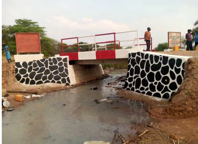
Bridge "Pont Fuke" at Fuke Village/ Kabalo after CFW activities – photo from end-line report
